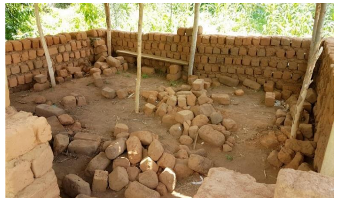
Figure 6. Incomplete, unsafe Reading Camp
